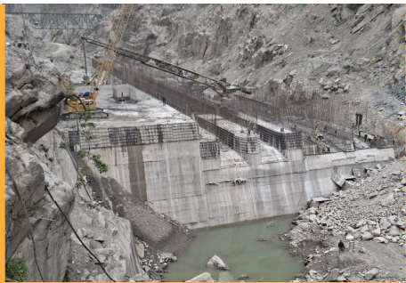
Kwar Hydropower Project in Jammu & Kashmir
