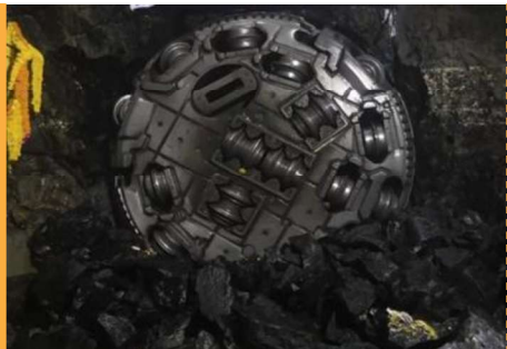
PG(RW) Water Tunnel Project in Maharashtra
