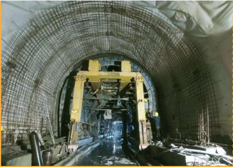
Tunnel T-7 Project in West Bengal & Sikkim
